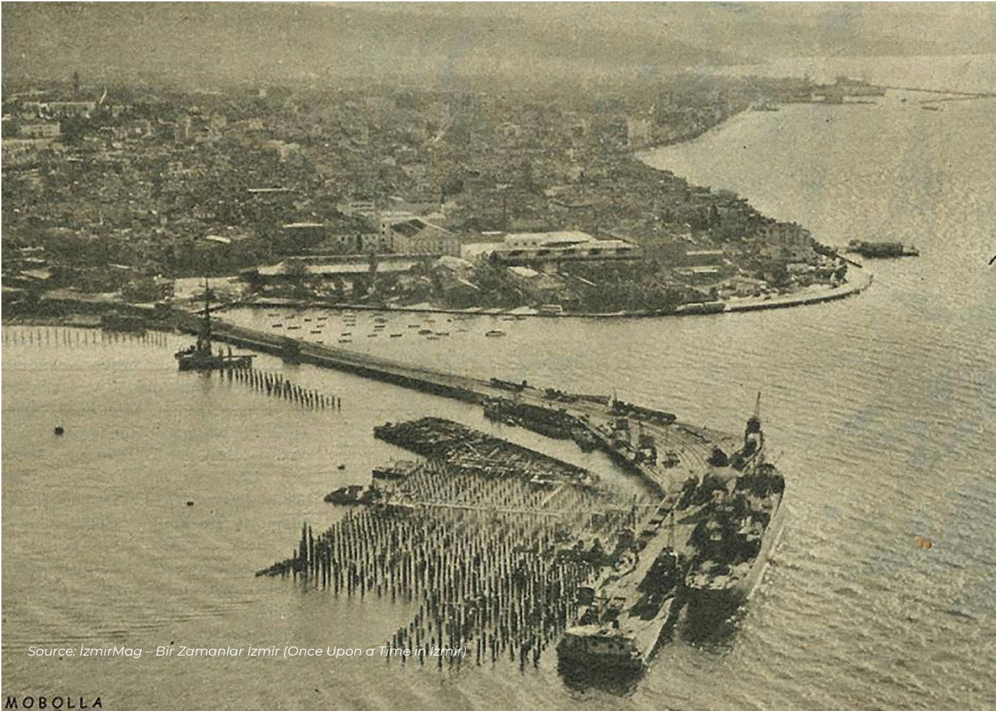
FIGURE 8. Construction of the TCDD Port of İzmir
