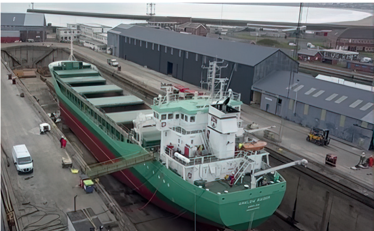
FIGURE 10. Dry-dock shipbreaking method
