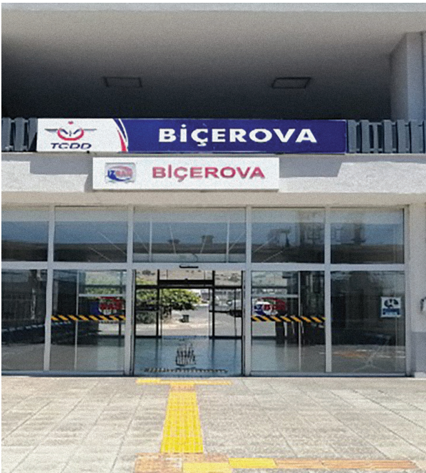
FIGURE 31. Biçerova Railway Station
