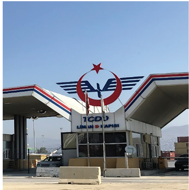
FIGURE 26. TCDD Port of İzmir Gate D
