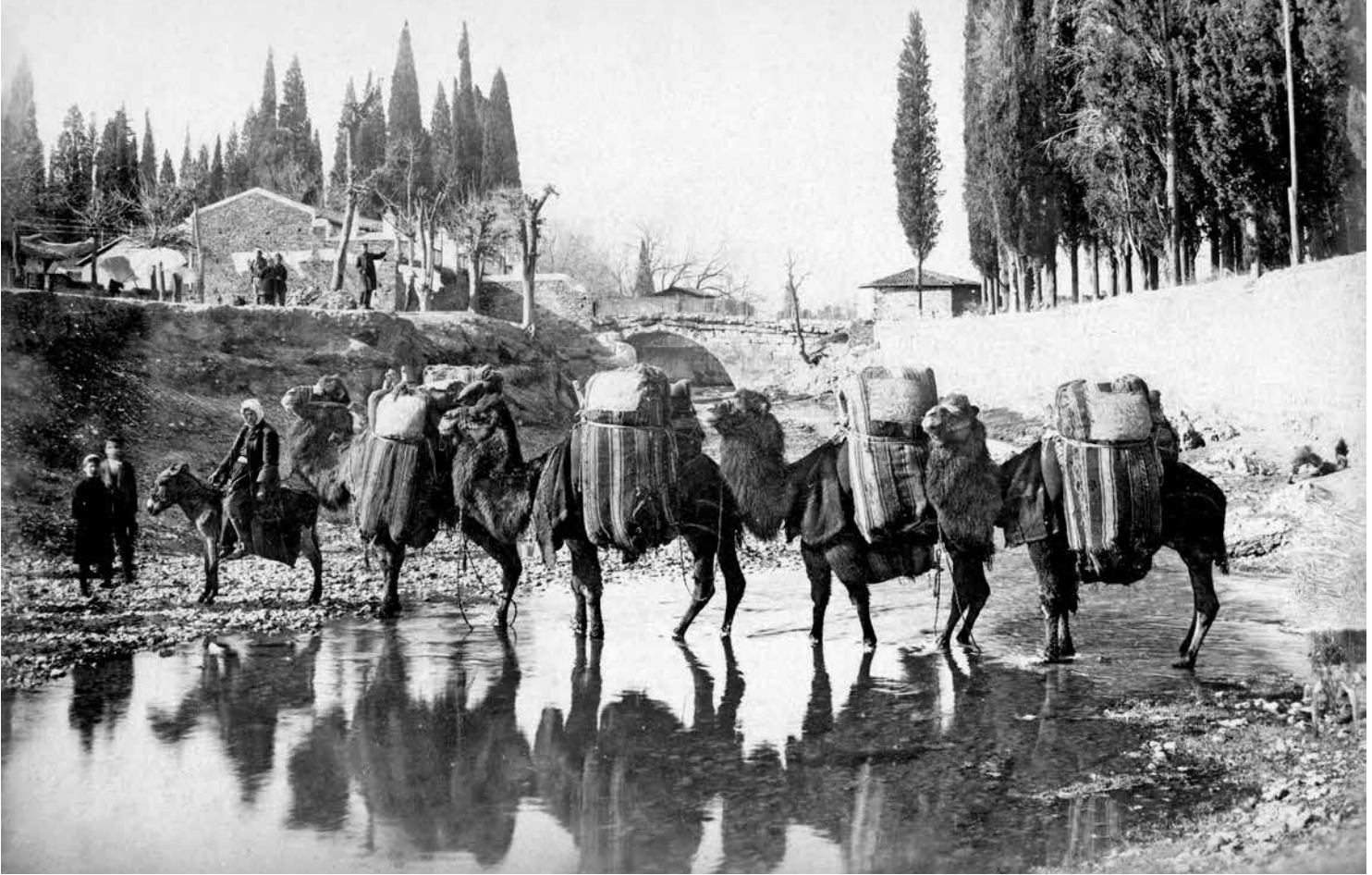
Kemer, Kervan Köprüsü, 1860-1870 ~ Anonim, Library of Congress
